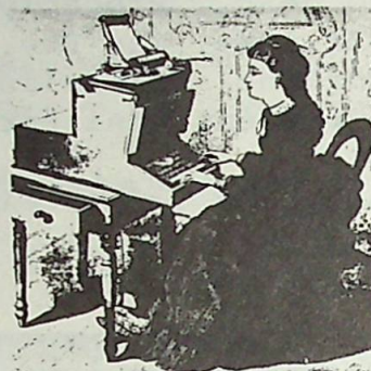
Sholes' writing machine (1868). Carriage was moved by foot pedals.
