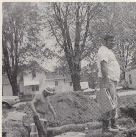
Raymond Snow and Don Whiteside building rest rooms for track
