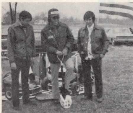
James Gamble, left and Bud Bullock, right, watch Johnny Parson, Jr. break ground for track.
